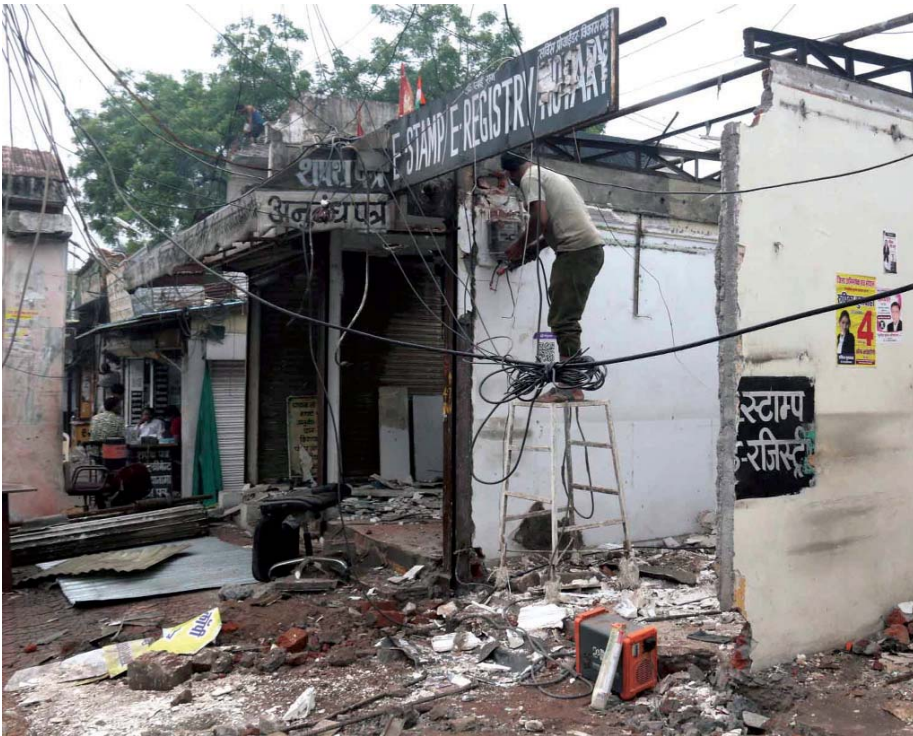
Stamp vendors and other shopkeepers remove goods from their shops as a road is widened under the Bhopal Metro Rail project near the old state assembly in Bhopal on Friday.
