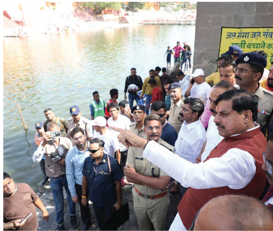
Chief Minister Mohan Yadav inspects the ongoing construction works in view of Simhastha: 2028 at Ramghat in Ujjain, Madhya Pradesh on Friday. Pioneer photo
